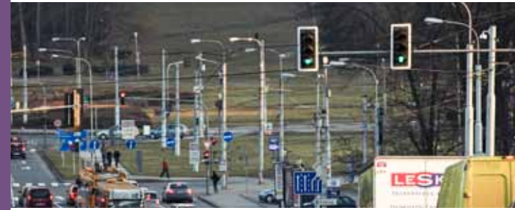
Adaptive Traffic Control and Public Transport Preference CROSS RS 4, eDaptiva Czech Republic, Zlín
